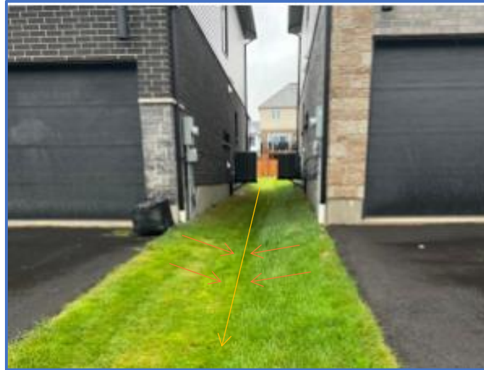
Common Property Line Drainage Swale
