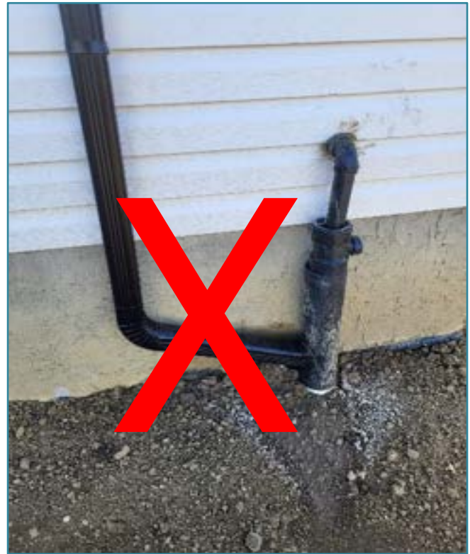
Downspout incorrectly connected to sump pump discharge
