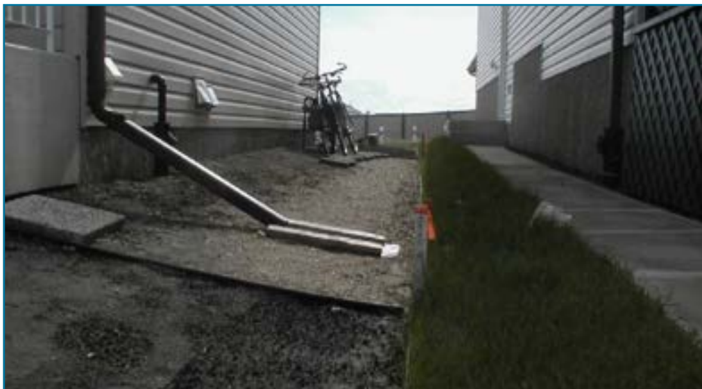
This rough grade base has been raised to match the final grade before placing decorative rocks. Ponding will potentially be minimized.
