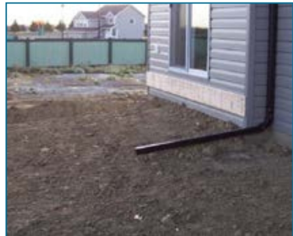
Slope Away From The Foundation Wall
