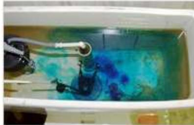
Wait 15-30 minutes. If the water in the toilet bowl changes colors, the flapper valve needs to be replaced. The flapper valve is located at the bottom of the tank; flapper valve kits are available at most hardware and home supply stores.
